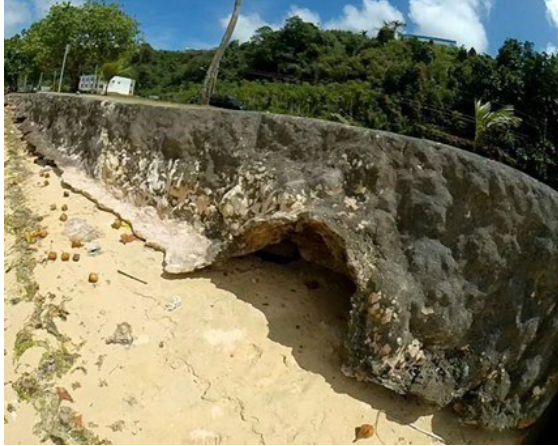
Figure 5. Voids where wall was constructed around trees that have since been removed or fallen
