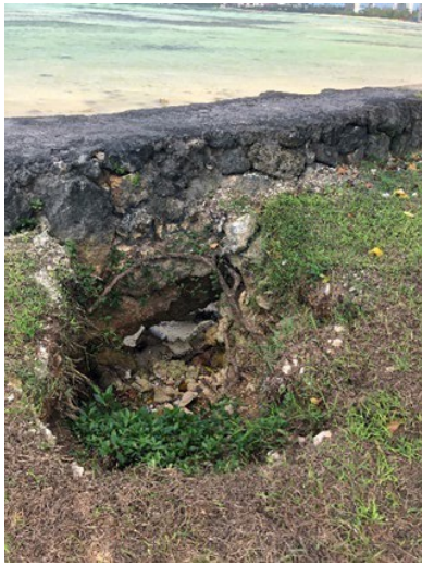
Figure 2. Sinkhole along landward side of wall in backfill
